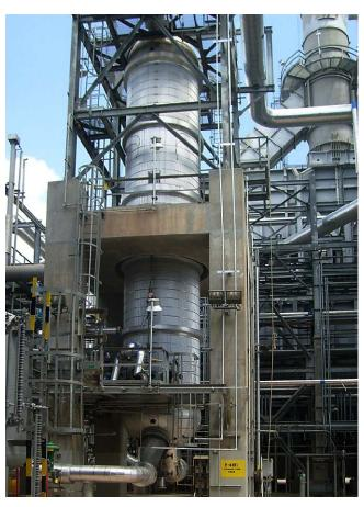
Packinox heat exchanger installed in a catalytic reforming unit.
